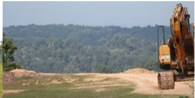
Bulldozer busy removing layers of sand and gravel
