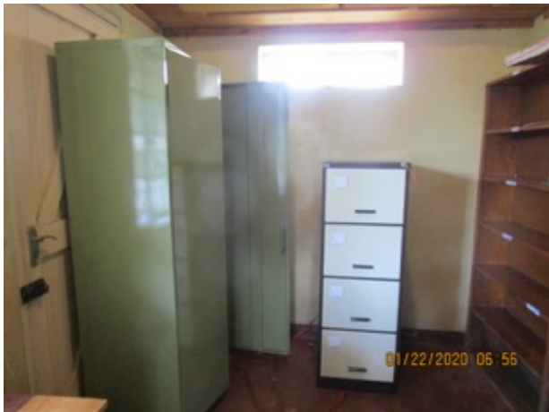
Fitting cabinets into the small archive room
